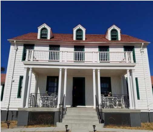
Vandenberg Air Force Base, The Boat House
